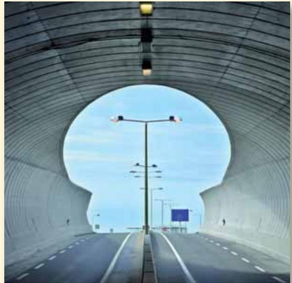
The concrete strength B65 has environment class 4 for construction, the timbers are FSC certified and the metal parts are made of aluminum and stainless steel. For the dimensioning of the complex form design a 3D model was developed. From this model the construction was further detailed and the specifications were set.
