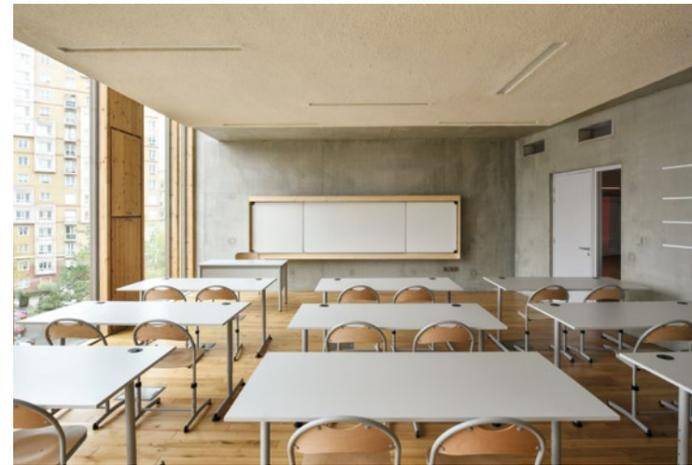
walls create unfolding sequences of compression and release along the routes. The plan varies from floor to floor, so the poured-in-place concrete walls do not vertically align, and loads are transferred through the slabs. Such irregularity is typically expensive, but the building was relatively economical at \$200 per square foot.
