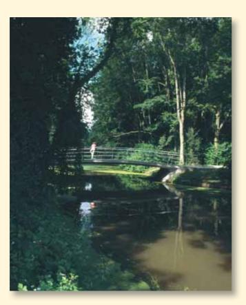
The lines of the landscape flow into the lines of the bridge. The bridge appears to grow naturally from the landscape, but retains its own identity. While the structural requirements, load figures, production restraints, maximum inclination, and minimum headroom all contributed to the final shape of the bridge, it remained important to maintain the flowing lines, the tension in the bridgehead lines, and the slenderness of the centre section.
