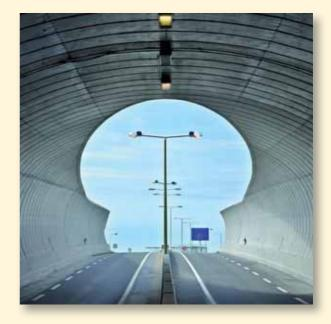
The concrete strength B65 has environment class 4 for construction, the timbers are FSC certified and the metal parts are made of aluminum and stainless steal. For the dimensioning of the complex form design a 3D model was developed. From this model the construction was further detailed and the specifications were set.
